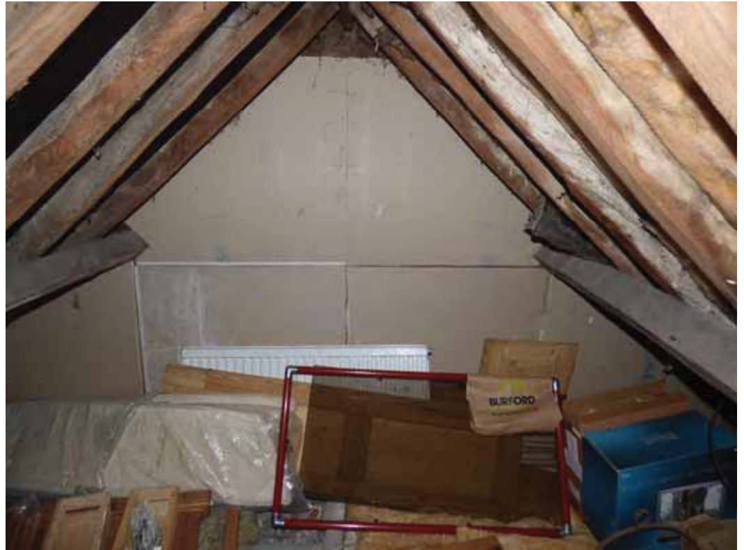
The better plasterboard faced wall to the left side room.
