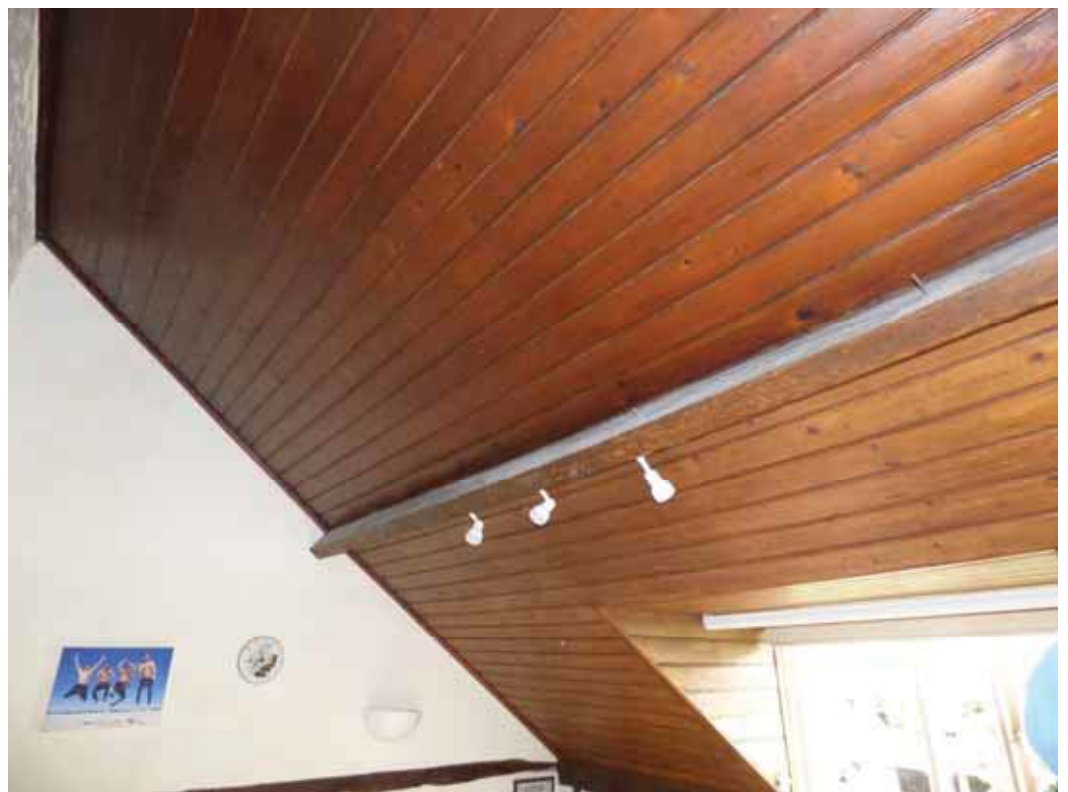
The boarded ceiling in the central rear bedroom.
