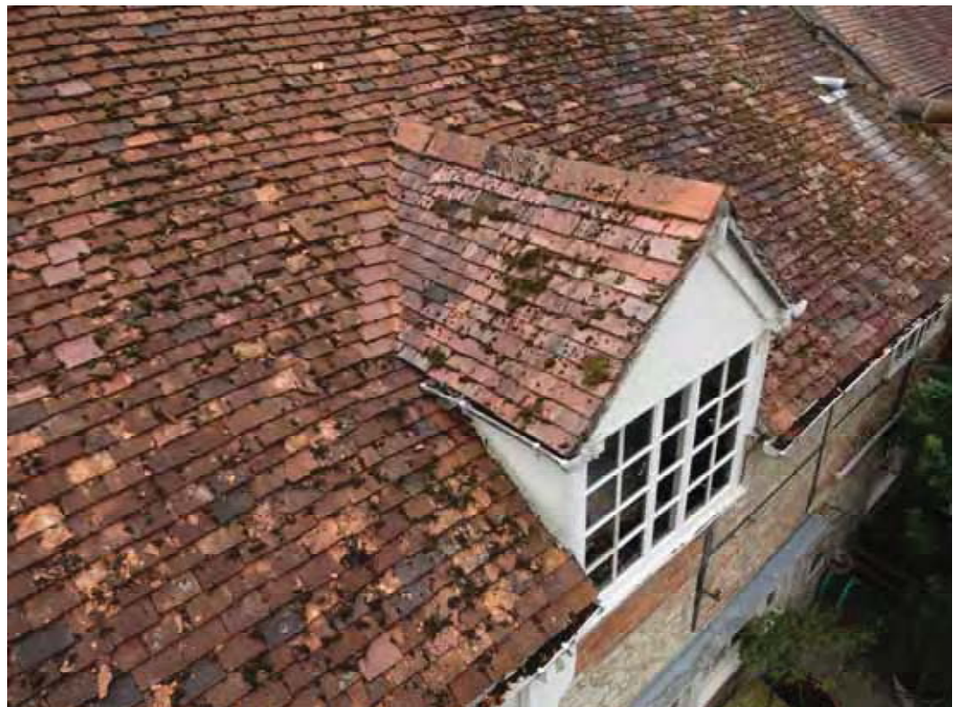
The right side slope.
