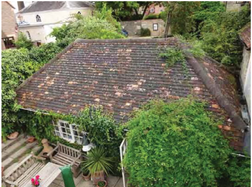
The extension roof.
