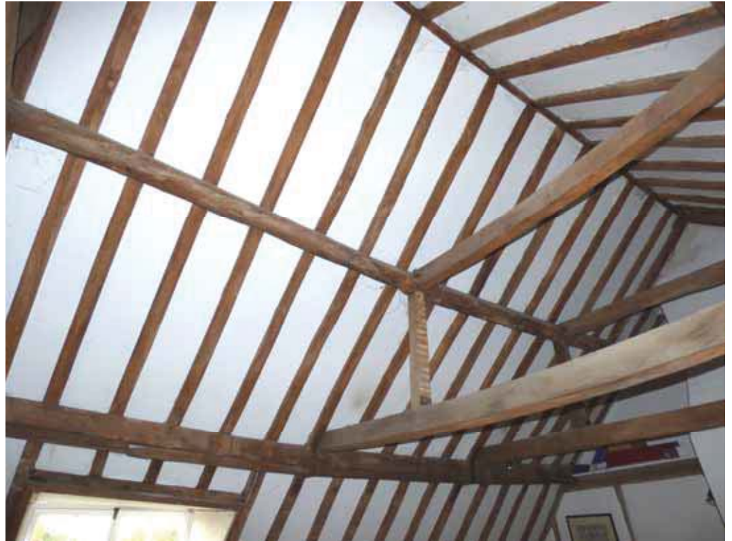
The front left side slope.
