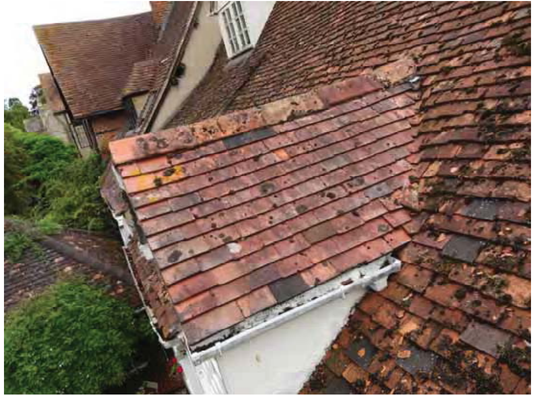
The left side roof slope.
