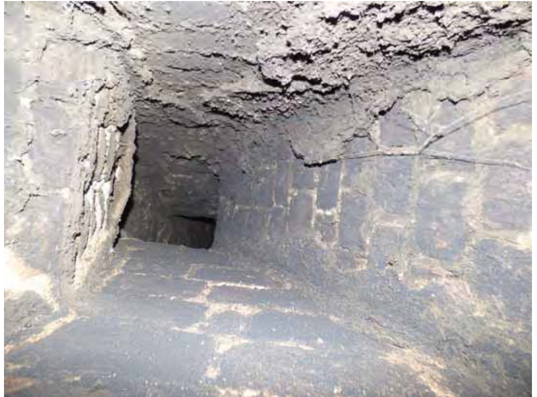
Internal view of the flue.
