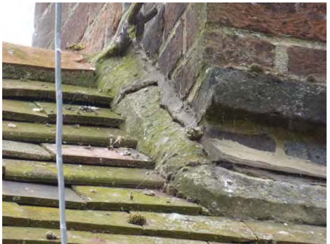
Close views of the basic patching undertaken to the fillets.
