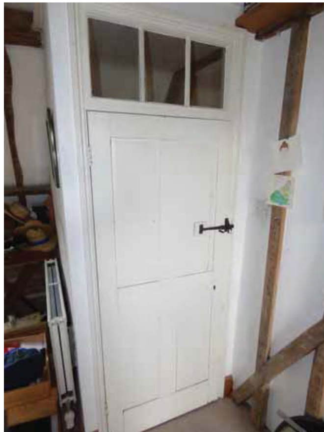
There are some good older panelled doors.
