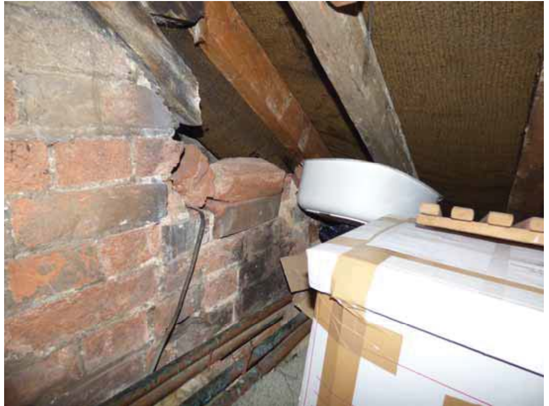
View left to the old stack.
