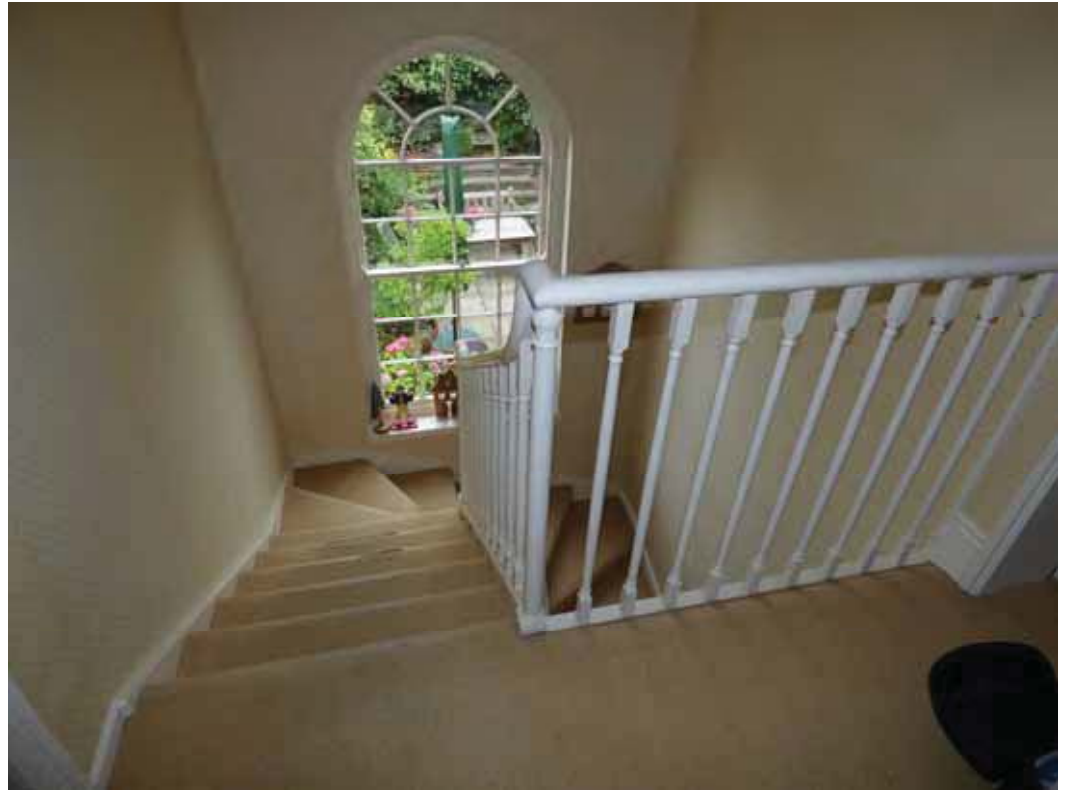
There is a good safe balustrade.
