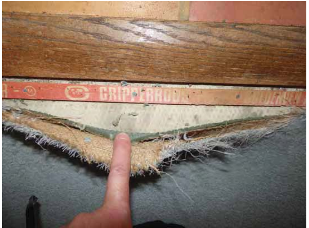
The exposed screed in the playroom.
