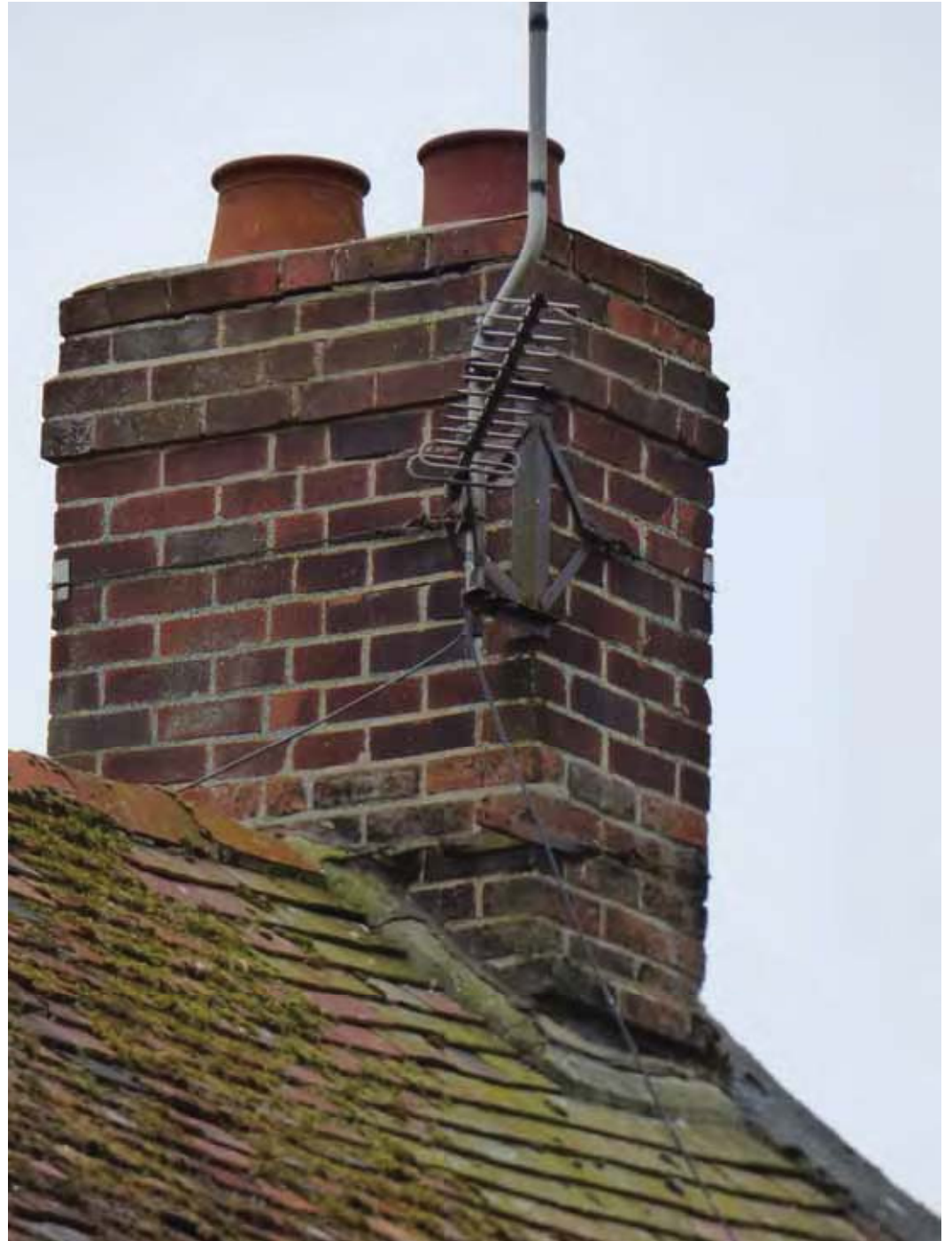
The rear right side view.
