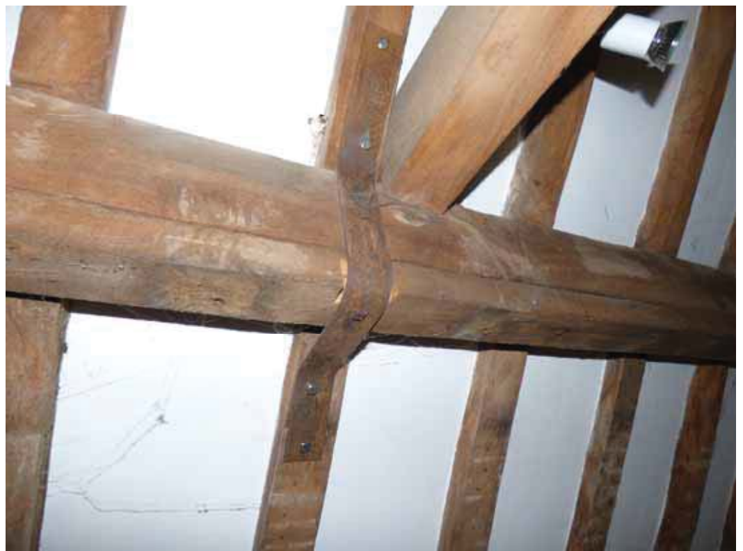
There are various straps and braces.
