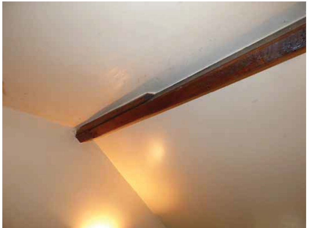
The purlin is visible within the room.
