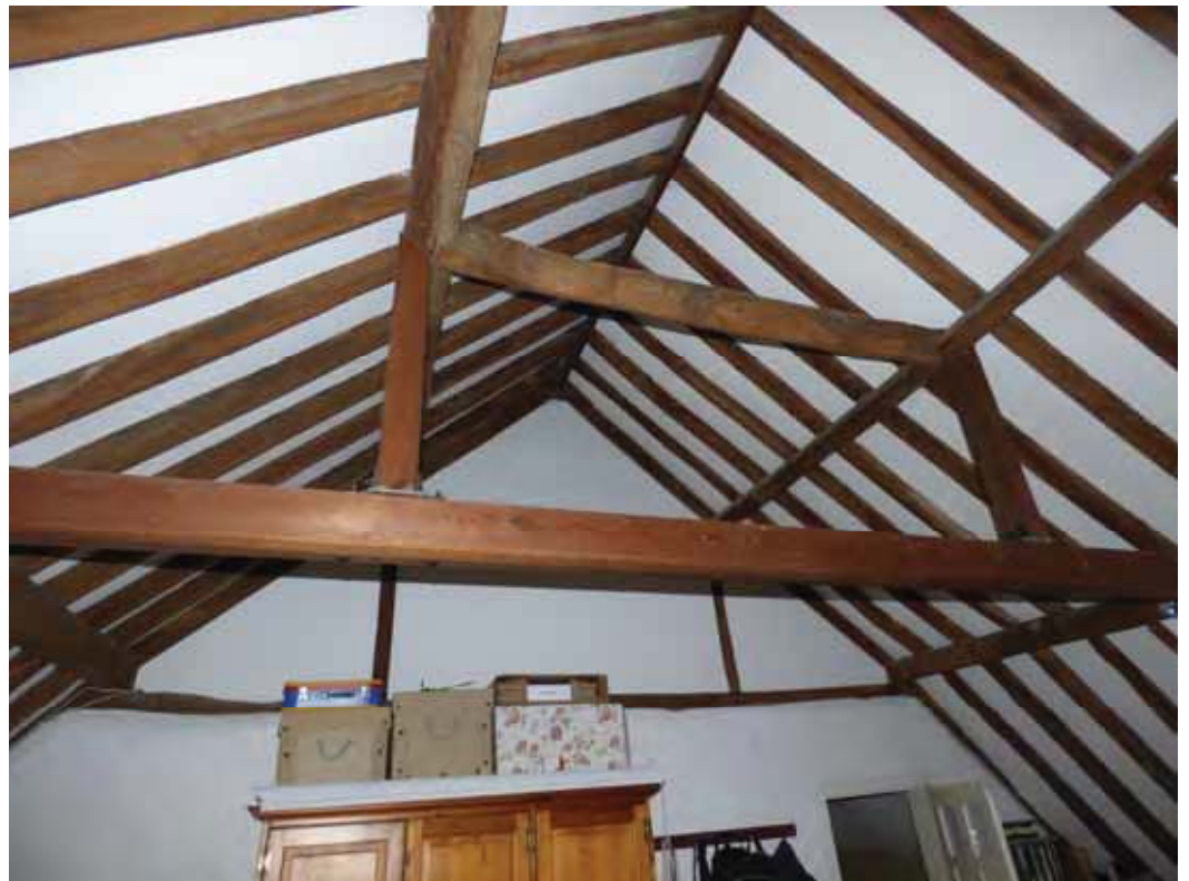
The right side and left walls.
