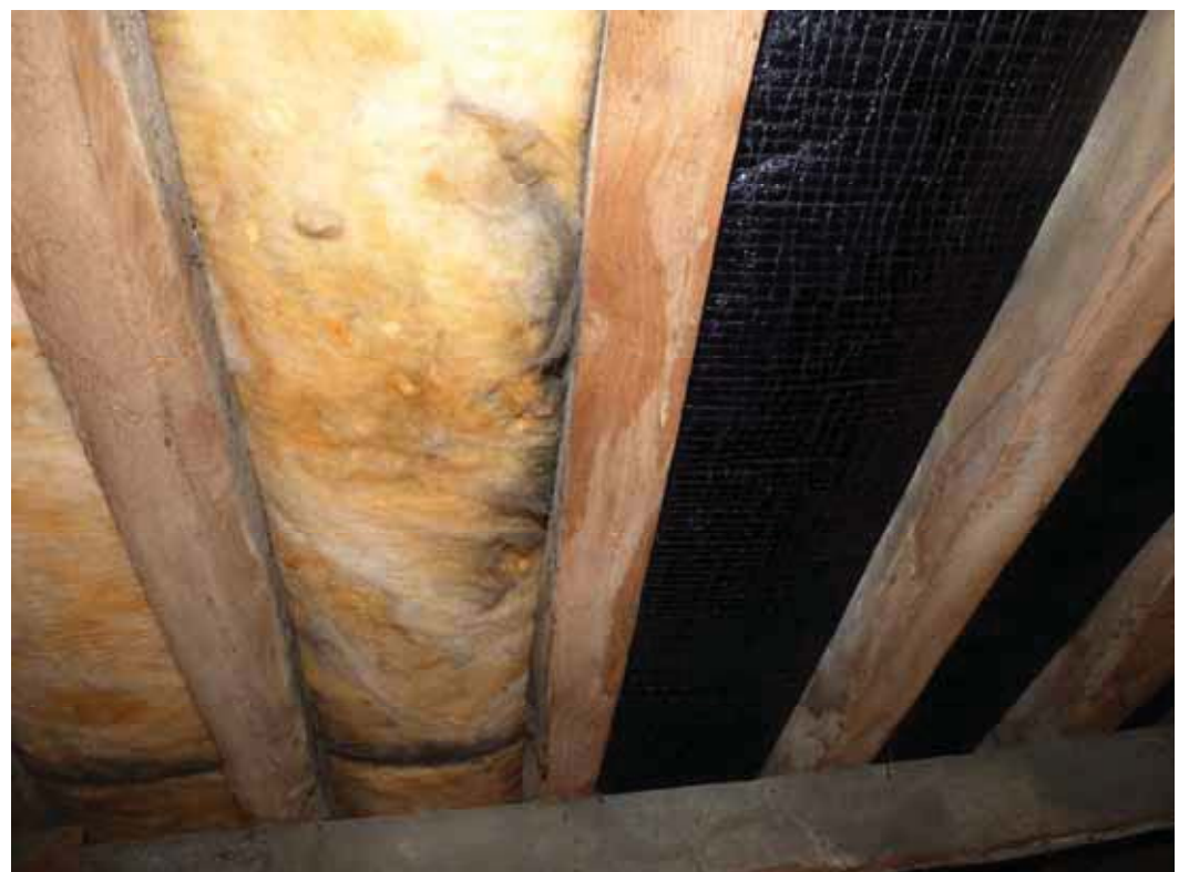
The roof slopes are lined with felt.
