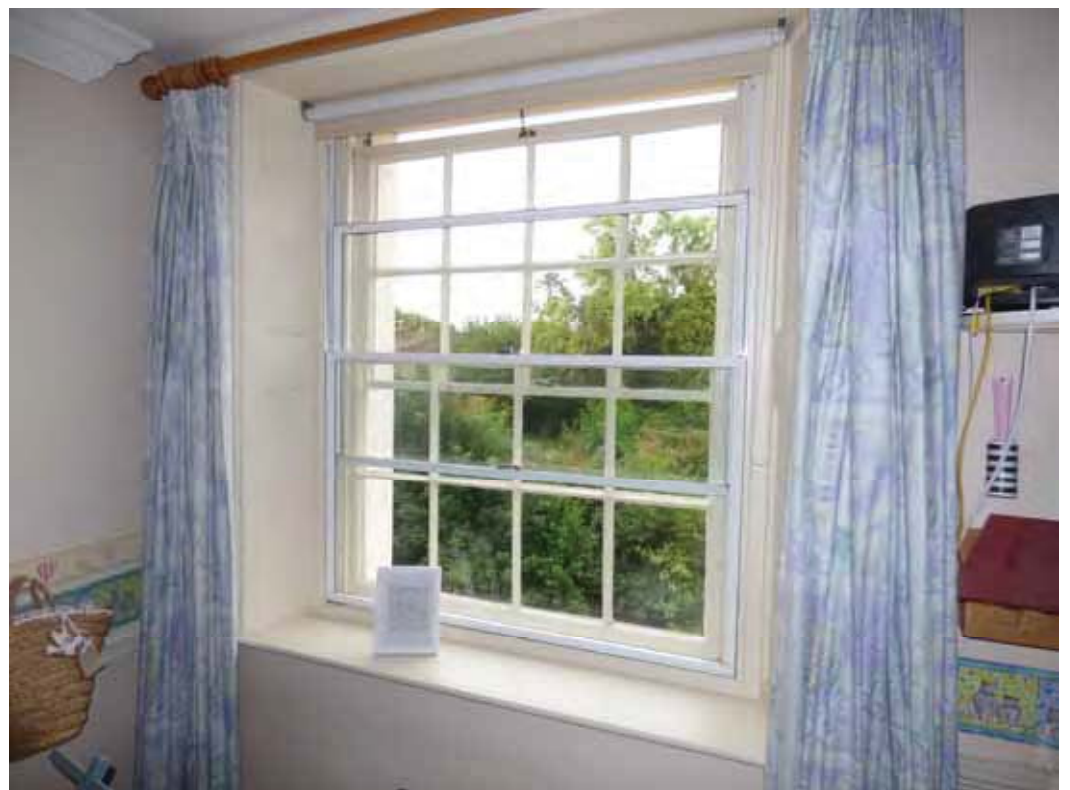
The house retains many older sashes.
