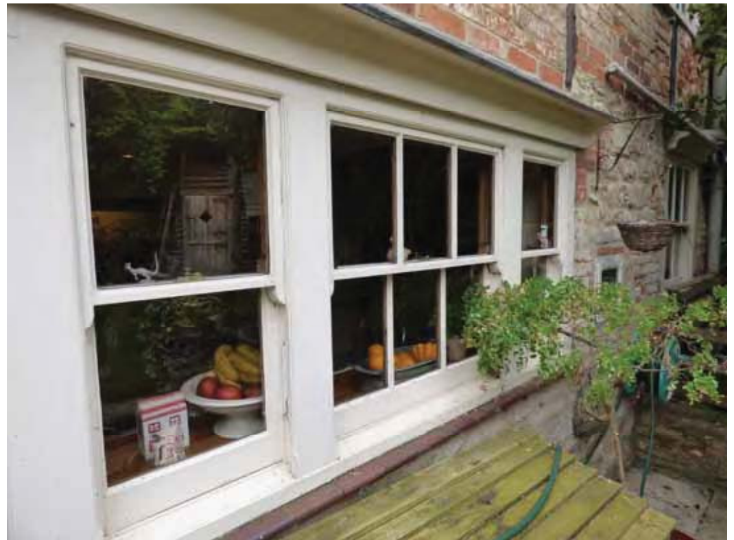
The relatively modern sash to the kitchen.
