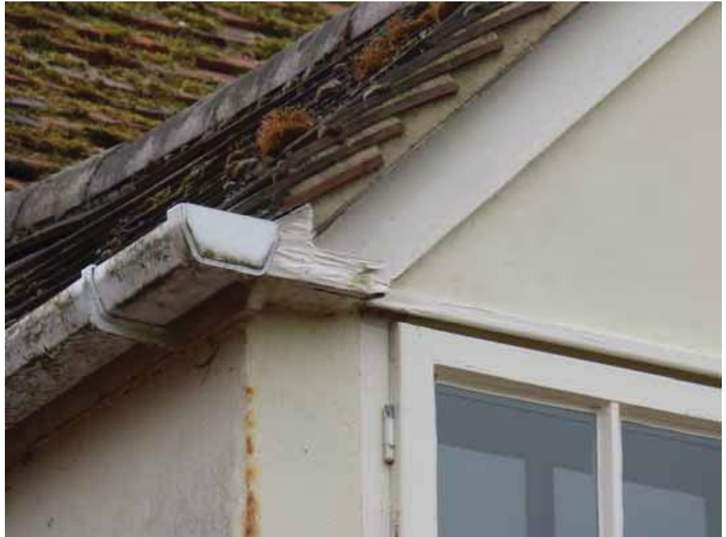
The other joinery timbers require patching and filling, prior to redecoration.
