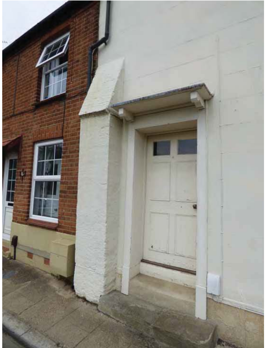
The buttress at ground floor level should help restrain movement.
