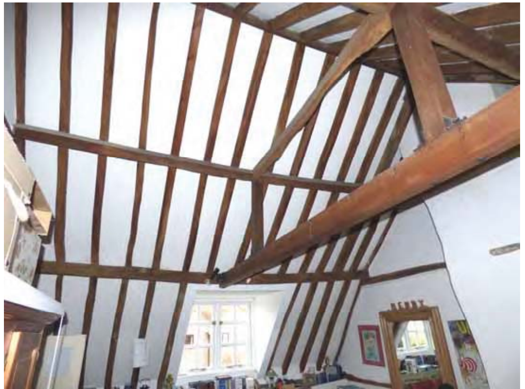
The front and rear slopes.
