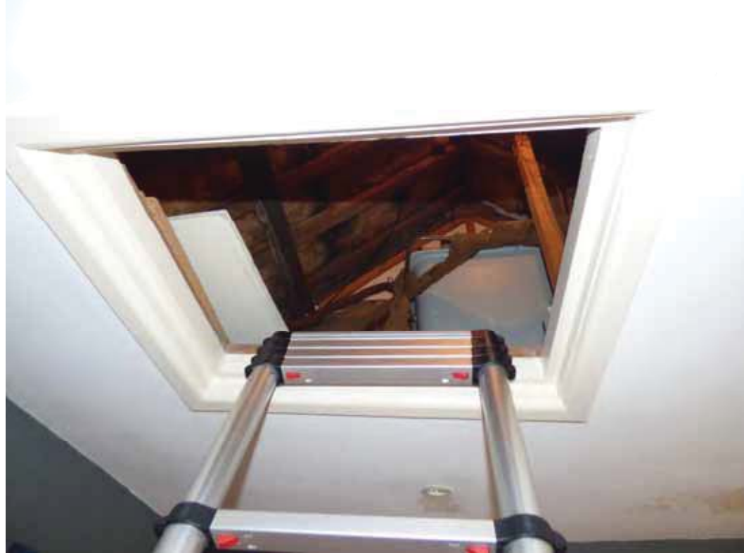
The access hatch into the main roof void.
