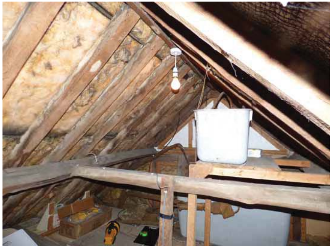
View to the rear right side slope.
