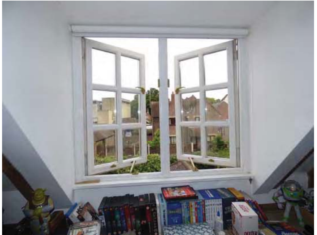
The newer rear window to the right side attic bedroom.
