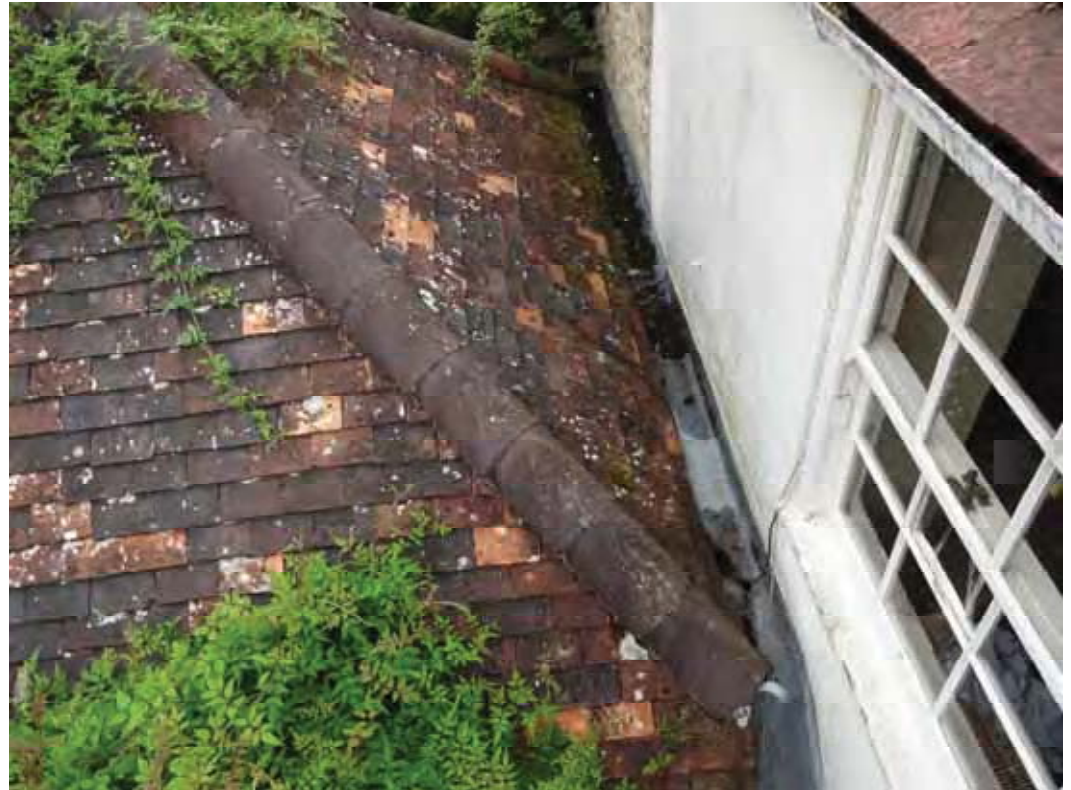
The front slope and lead lined valley gutter.
