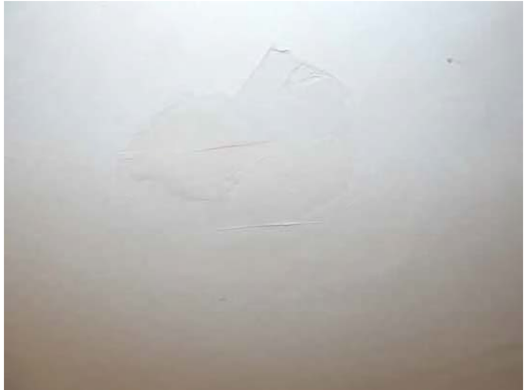
The finishes are basic in areas and would benefit from upgrading.
