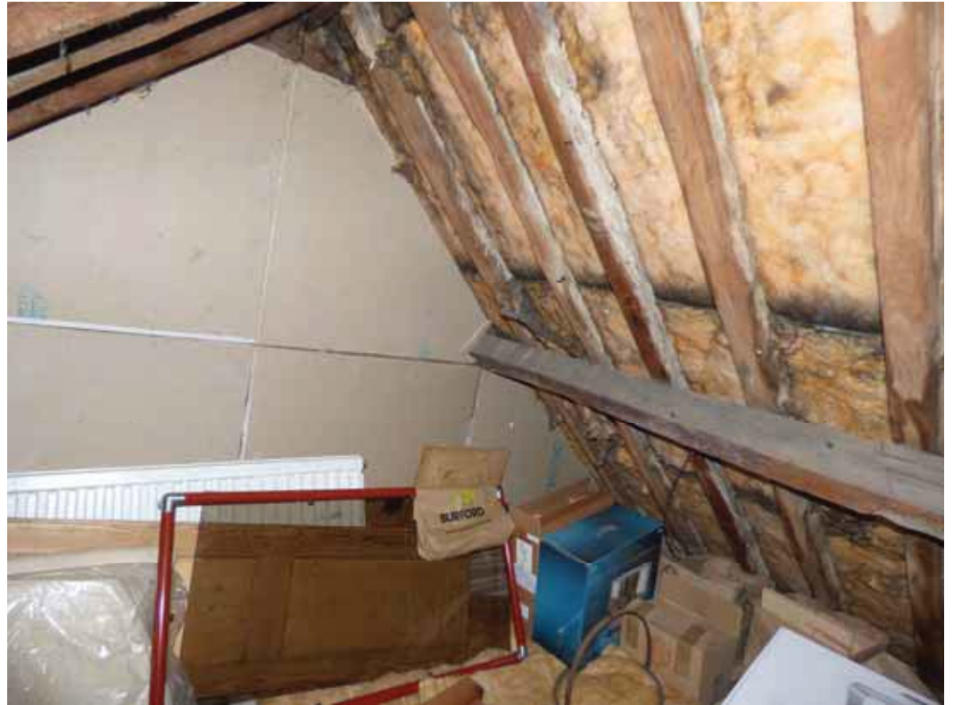
View to the rear left side slope.
