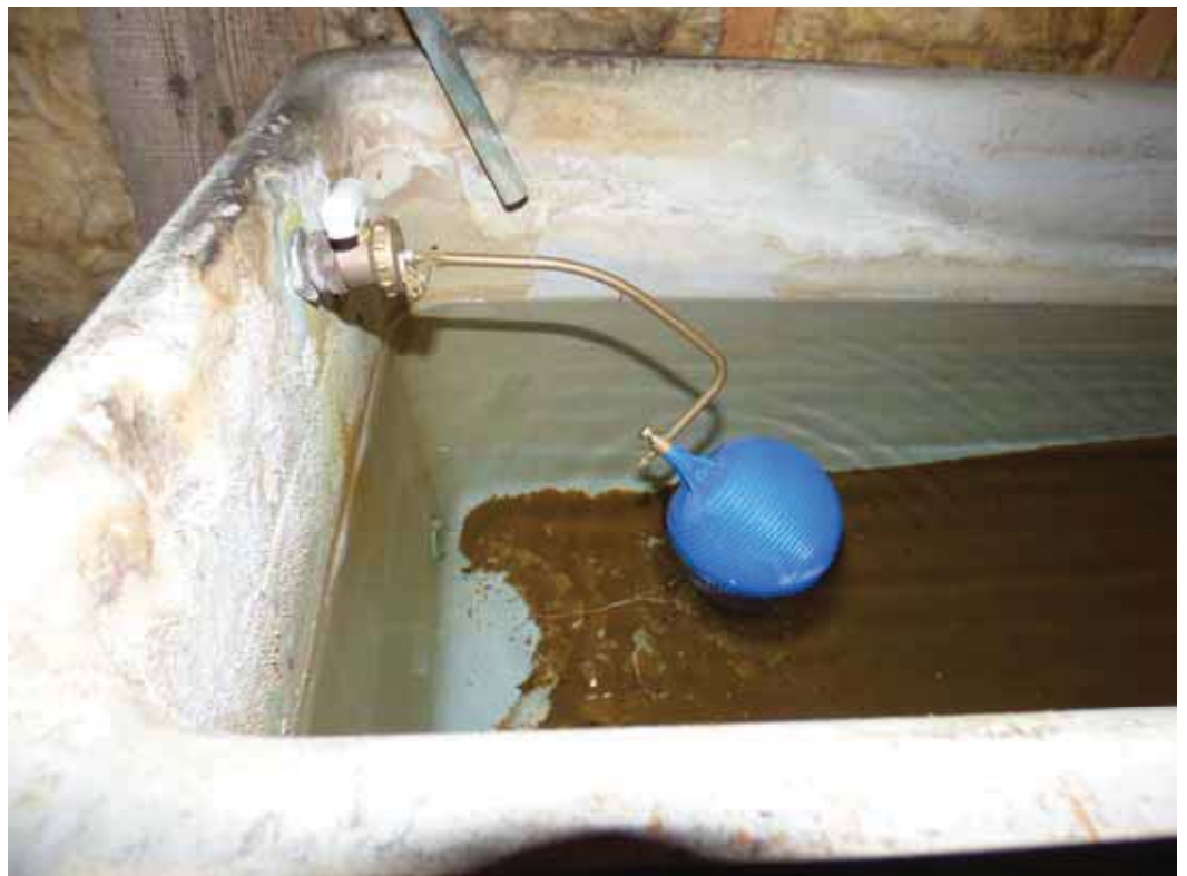
Internal view – the ballcock has been renewed.
