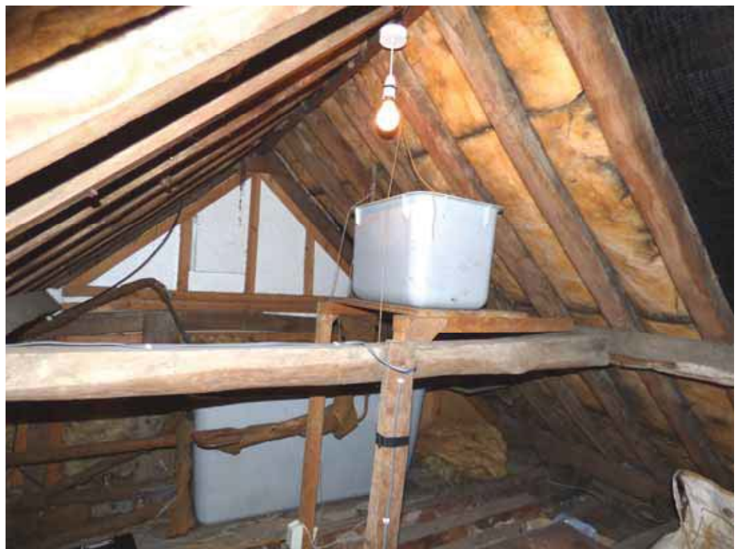
View to the front right side slope.
