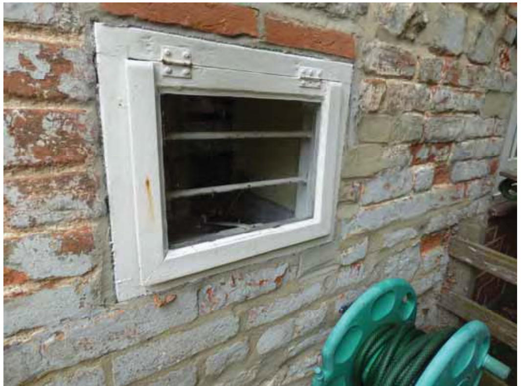
An old painted-up casement to the kitchen.
