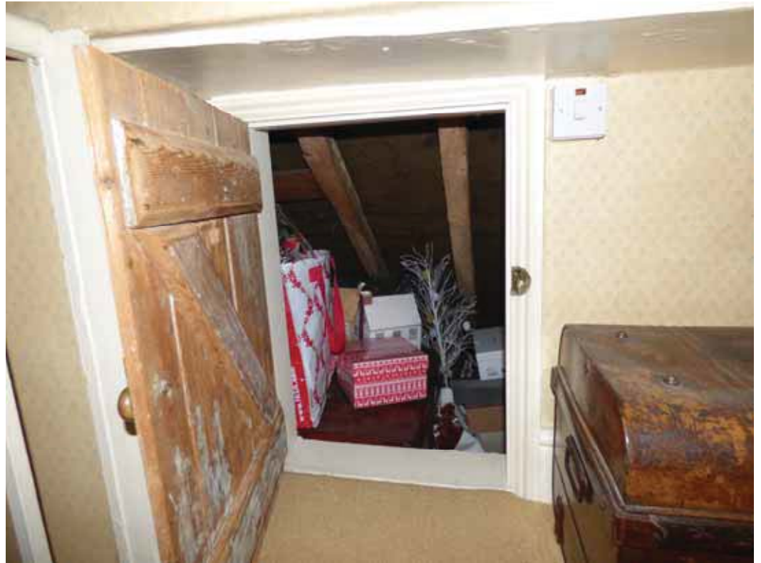
There is limited access to the rear eaves.
