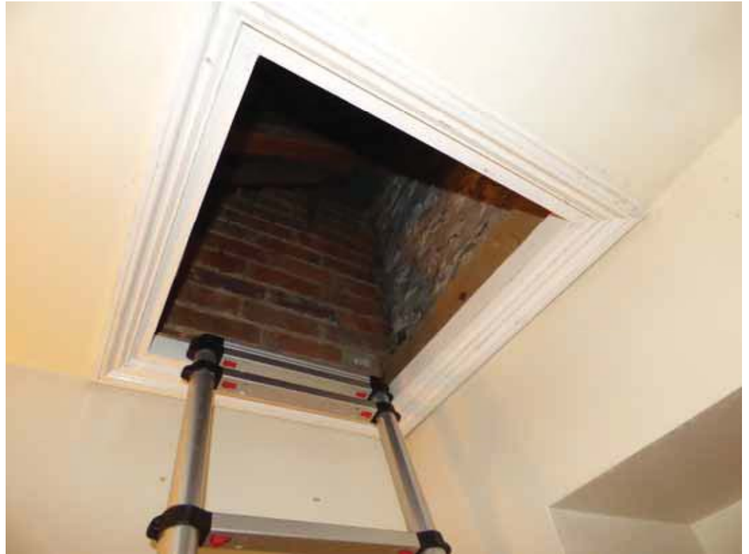
There is access to the eaves void over the shower room.
