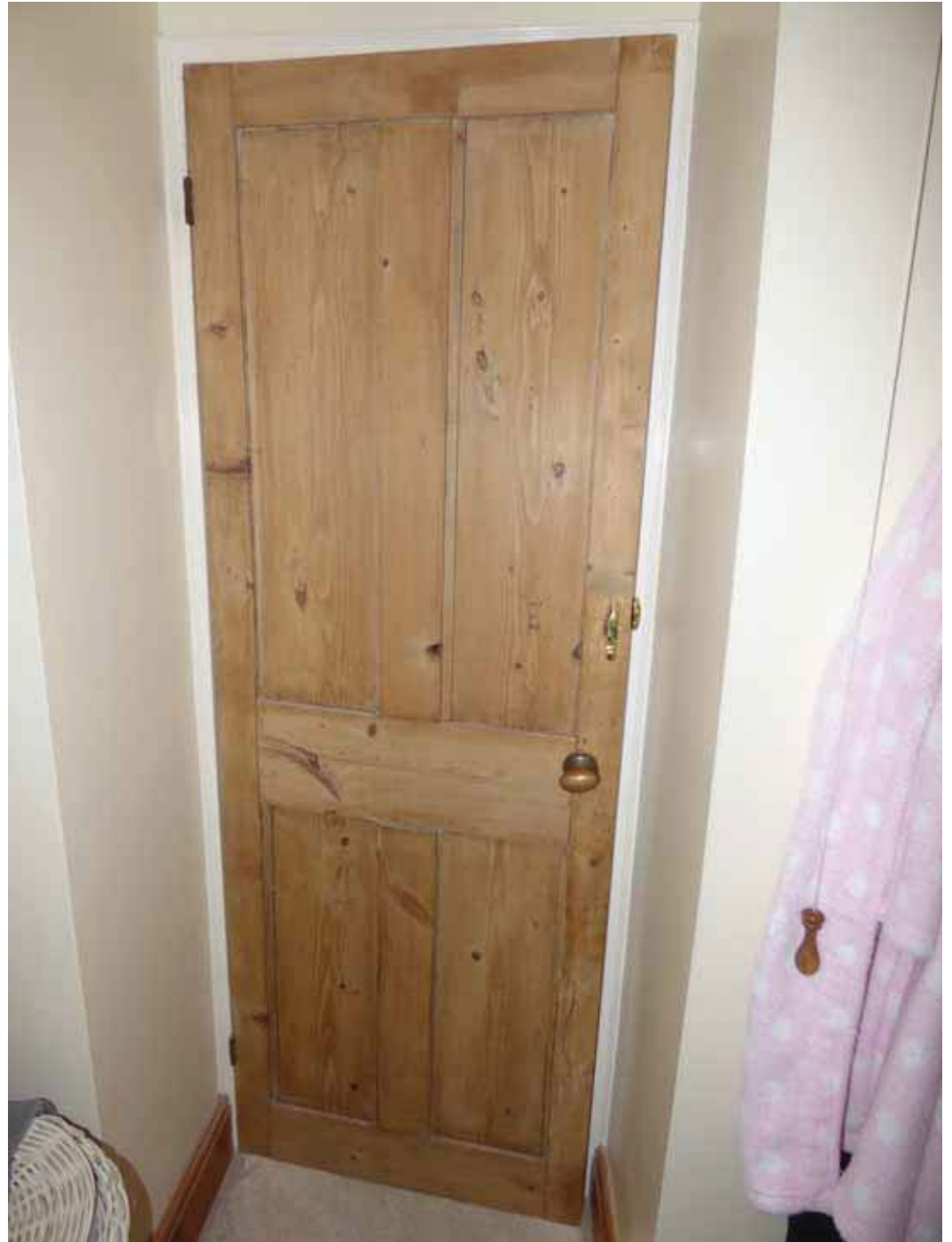
Some doors have been stripped – a finish popular with purchasers.
