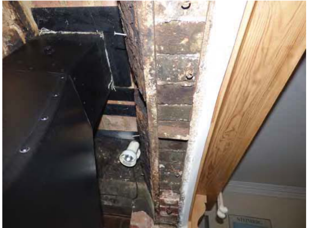
The brick arch supporting the opening is satisfactory.
