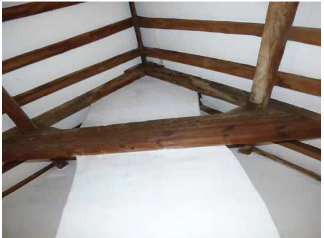
Internal view of the chimney breast.
