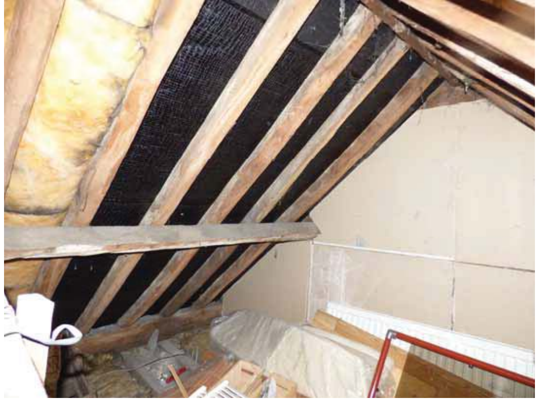
View to the front left side slope.
