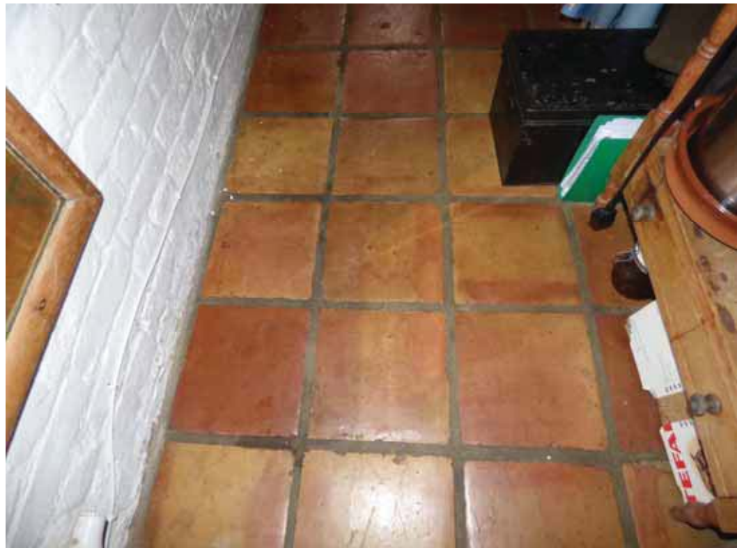
There are tiled finishes.
