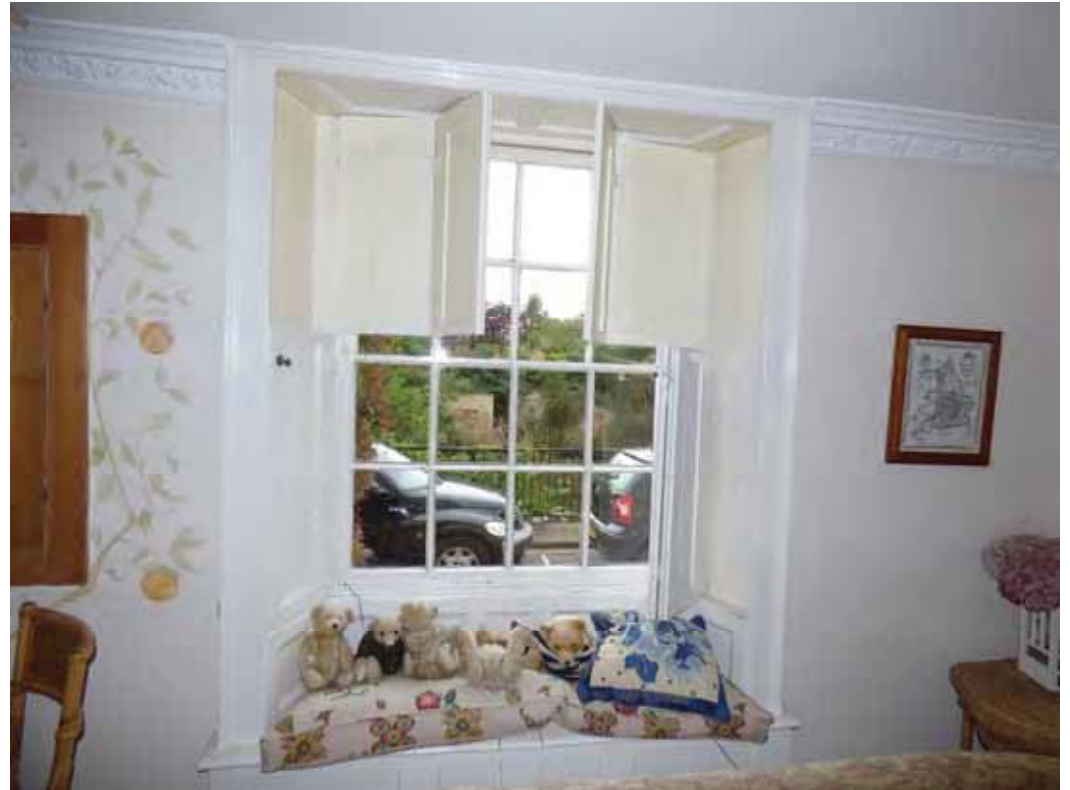
Some frames retain shutters.
