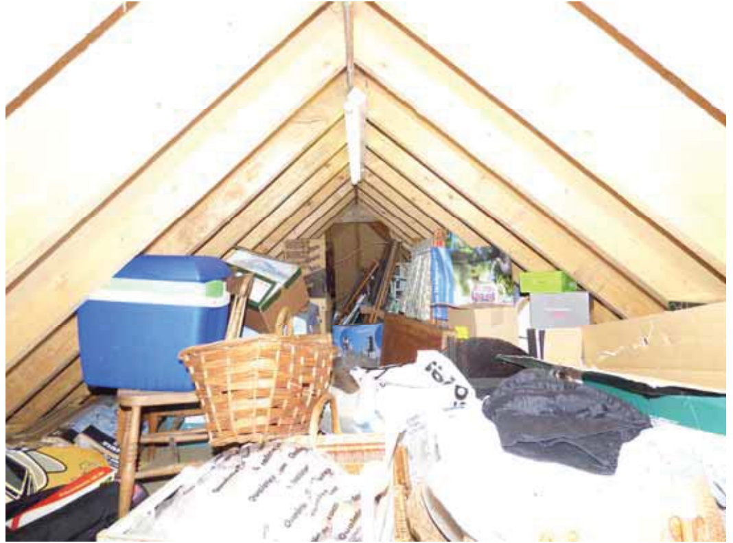
View to the front – the loft provides good storage, but should not be overloaded.
