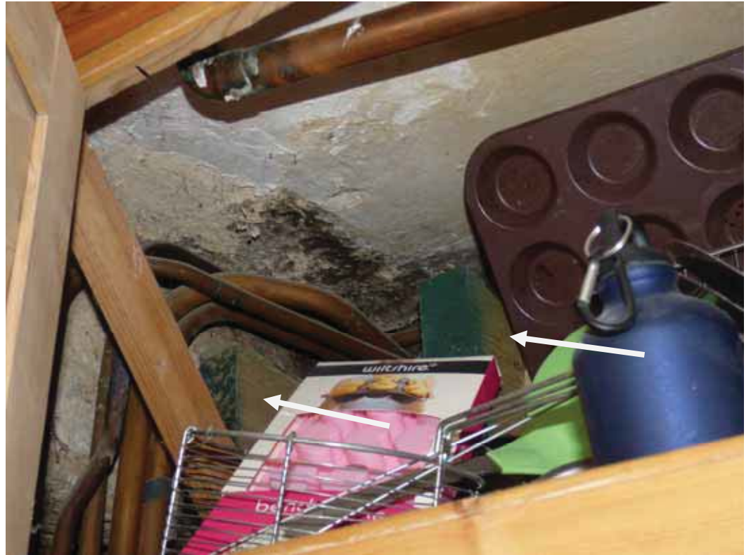
The older floors are considerably off-level, but some new joists have been installed – these support the shower room floor.
