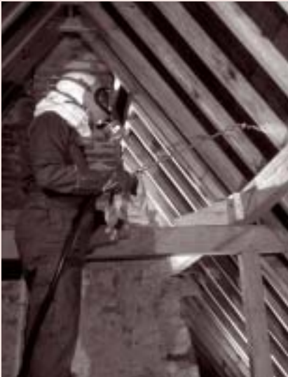
Remedial timber treatment with permethrin
